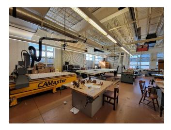
Lighting in most of the building is fluorescent fixtures. Most of the spaces have recessed mounted fixtures. Lighting control is through wall switches. There were no issues noted with this system.
