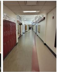
Walls are painted CMU, gypsum board and plaster. Wall finishes are in fair condition. There are sections of the original 1930 building where the plaster is in disrepair due to water infiltration/damage.
